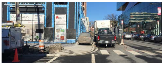
Figure 3 – Parking within encroachments.
