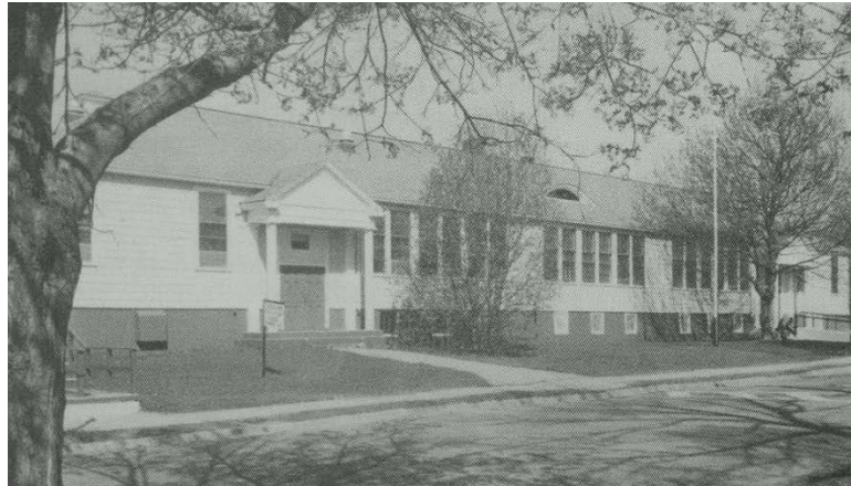
Figure 2: Findlay School building, 1993 (Image provided by Applicant)
