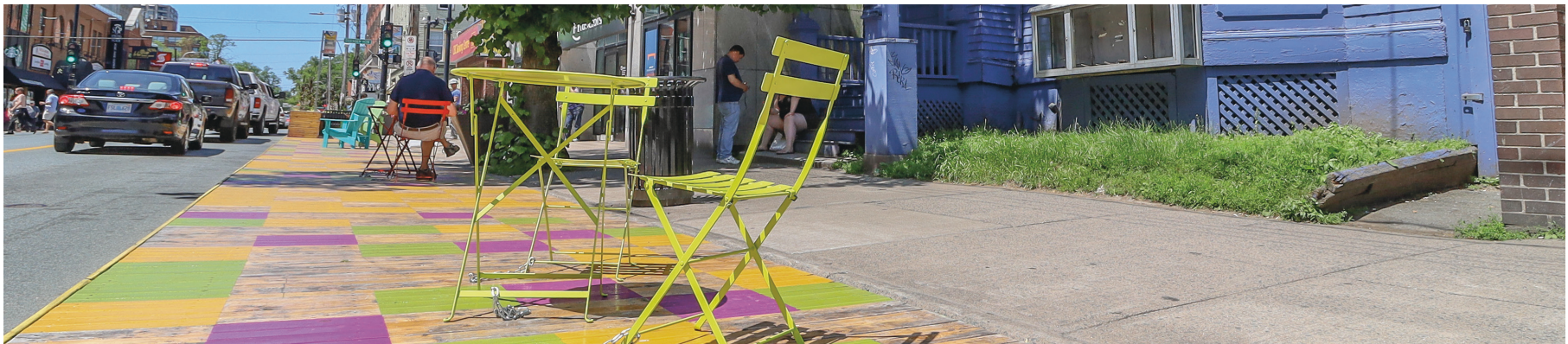
Example 2: Open space material and colour patterns in Imagine Spring Garden Road project reflect Spring Garden Road character.
