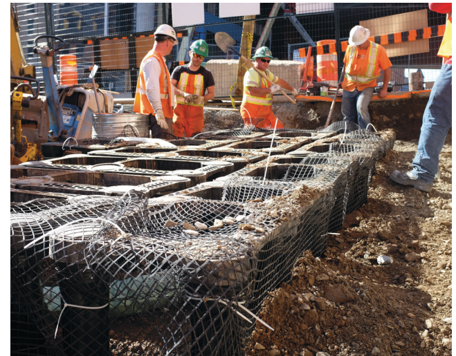
Example 3: Soil cells support healthy trees.
