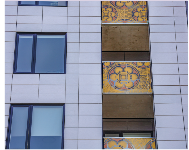
Example 2: Balconies reflecting historical context with materials and colour patterns.
