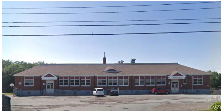
Figure 4: Flemming Tower School, 2018 (Google Maps)
