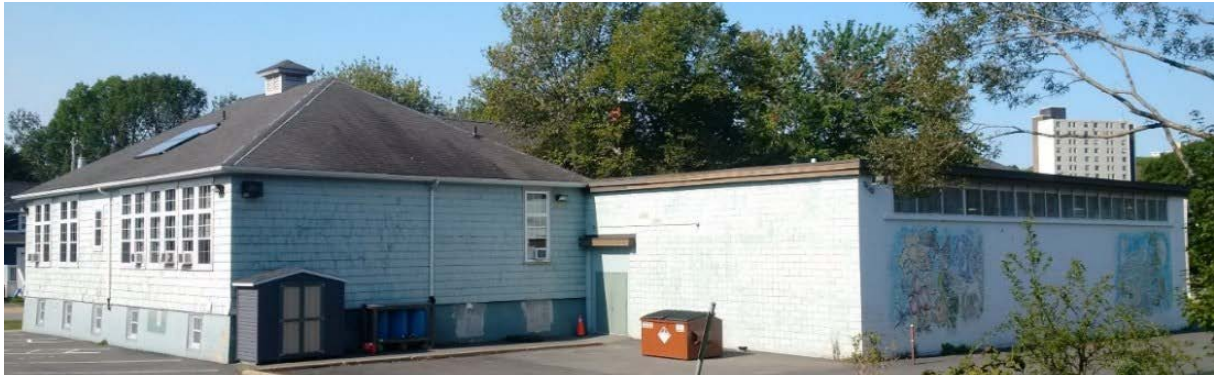
Figure 6: Rear gymnasium addition, 2018 (Photo provided by Applicant)
