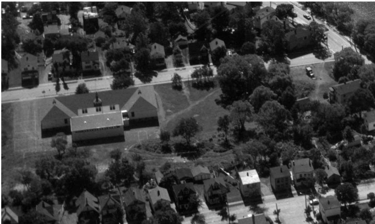
Figure 1: Aerial photograph of the Findlay School property, 1963 (HRM Archives)
