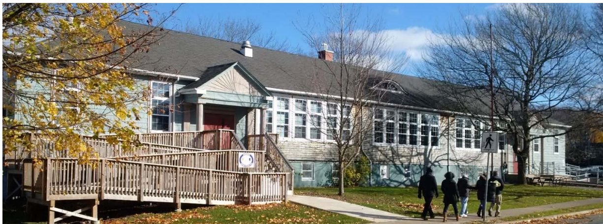
Figure 7: Findlay Community Center, 2018 (Photo provided by Applicant)
