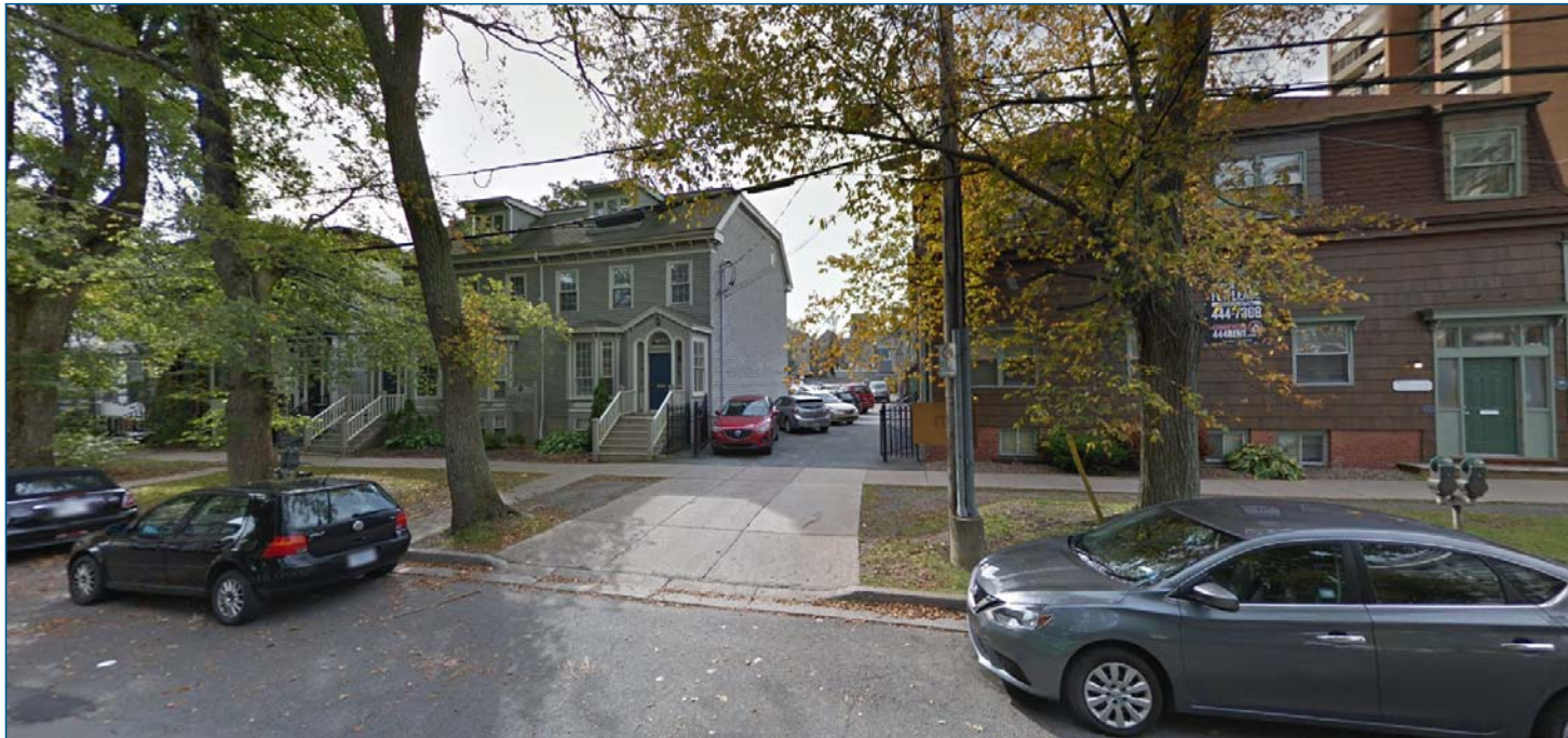
Subject site looking southwest from Carlton Street
