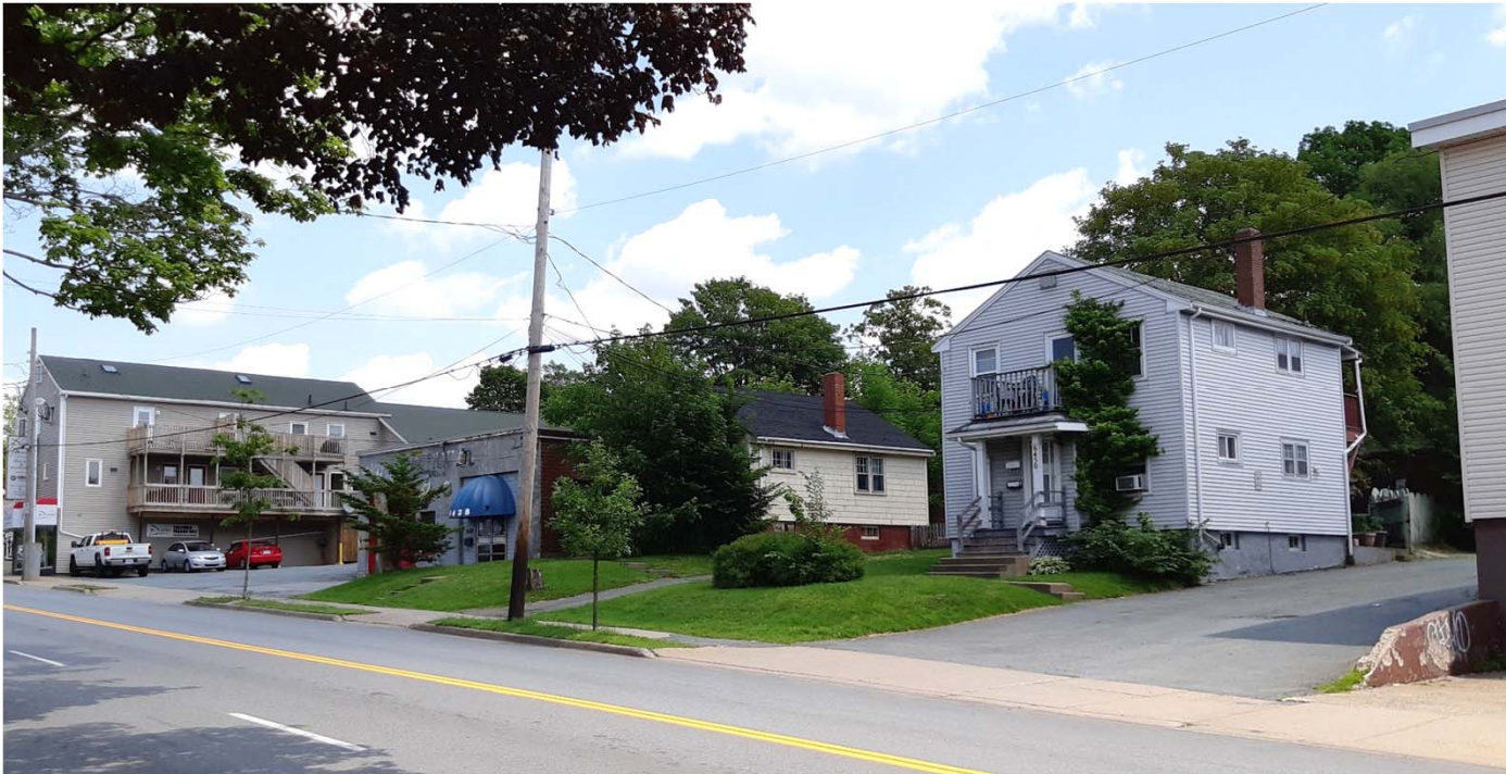
Subject Site (Near Northern Boundary)
