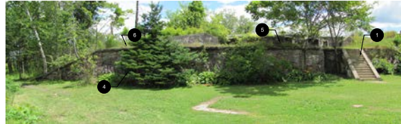
FRONT WALL - NORTH END
