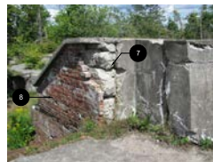
TELEGRAPH POST - FRONT OF WALL
