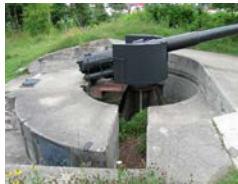
NORTH GUN EMPLACEMENT - GUN AND STAND TO BE REMOVED BY OTHERS
