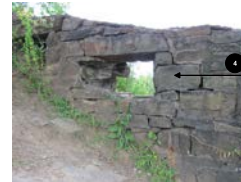
SW WALL LOOPHOLES
