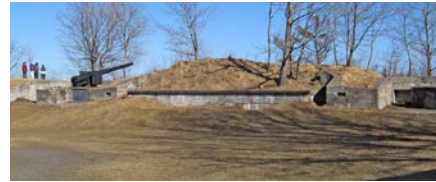
NORTH GUN EMPLACEMENT AND CENTER WALL
