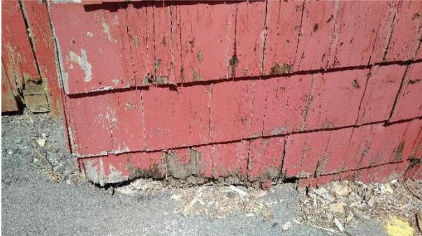
Figure 1: Deteriorated Siding
