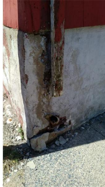
Figure 6: Foundation in Need of Repair
