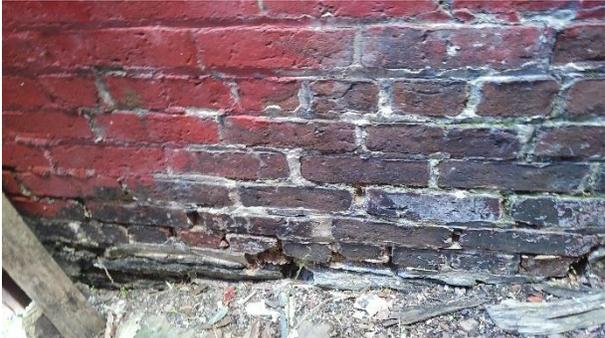
Figure 2: Brick Foundation in Need of Repair
