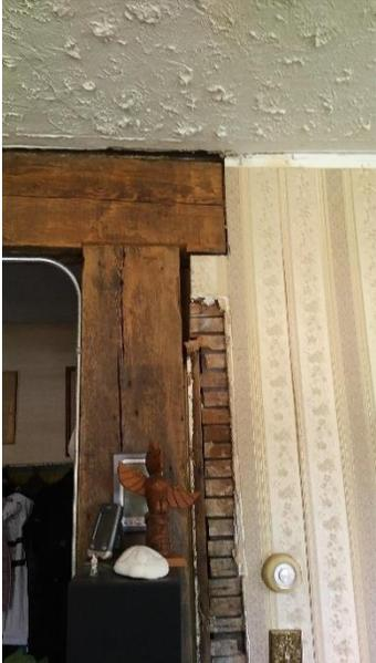
Figure 4: Wall Replaced with Post and Beam
