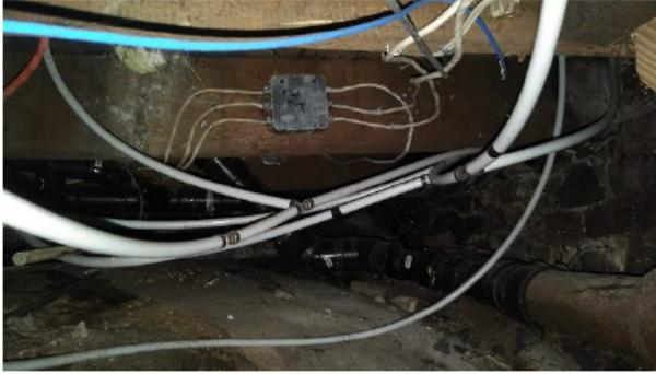
Figure 5: Wiring in Uninsulated Crawl Space
