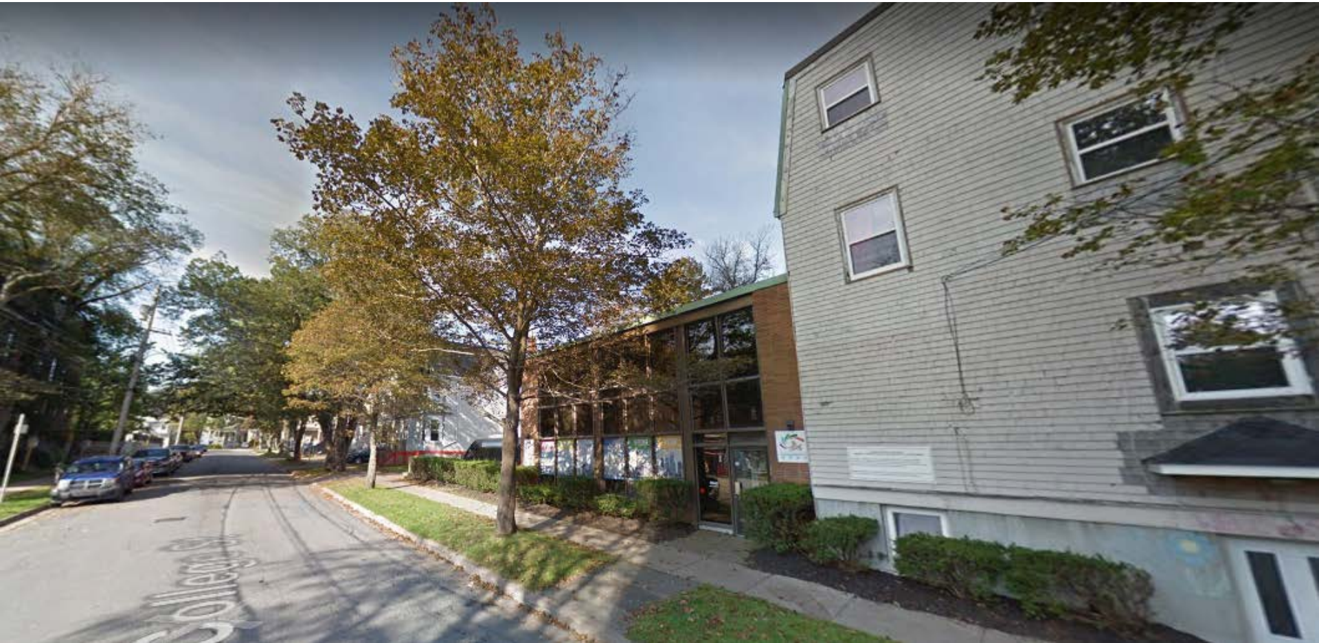
Subject site looking west from College Street.
