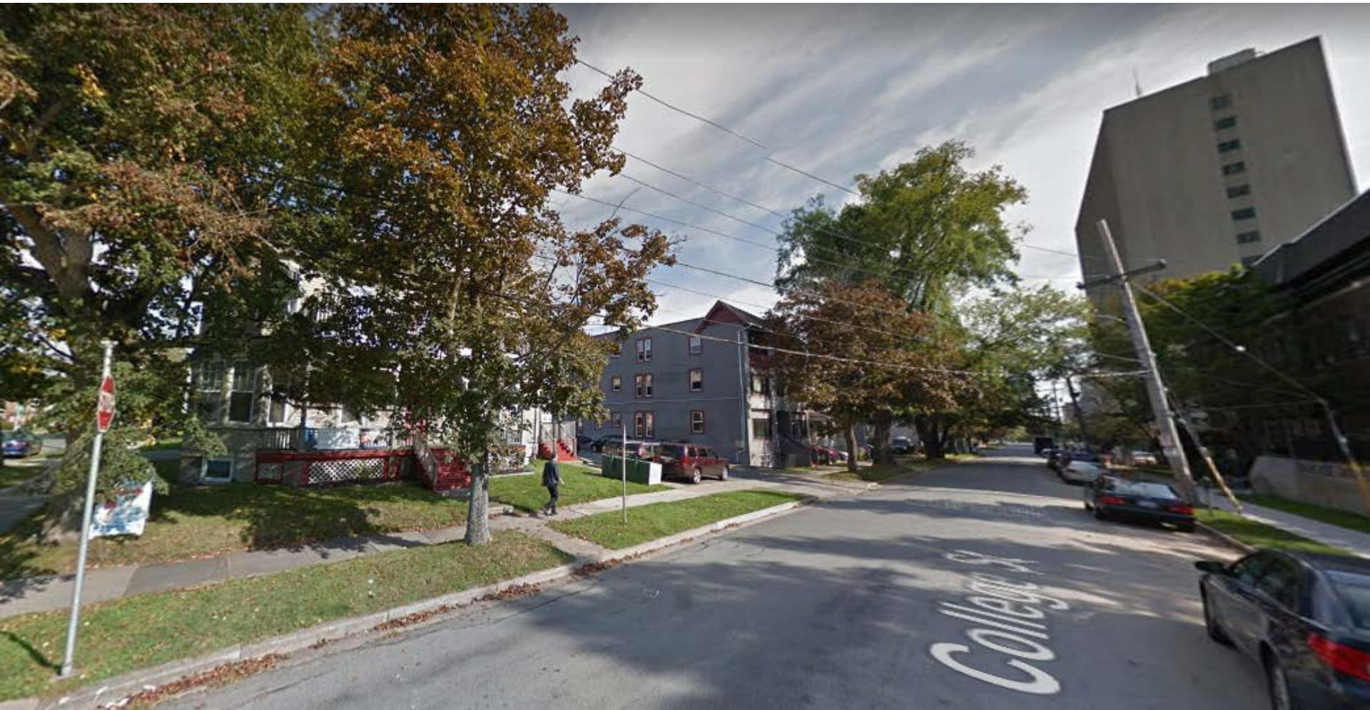
Subject site looking northeast from College Street.
