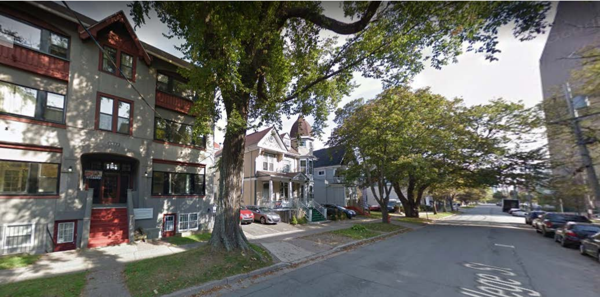
Subject site looking northeast from College Street.
