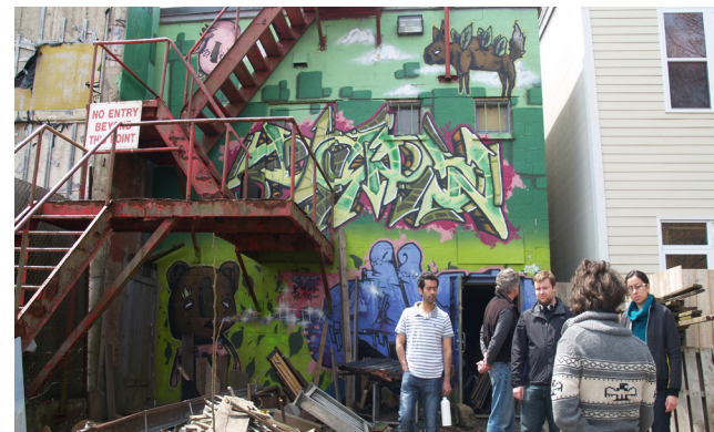
2014 Rear access to the theatre (before new fire escape)
