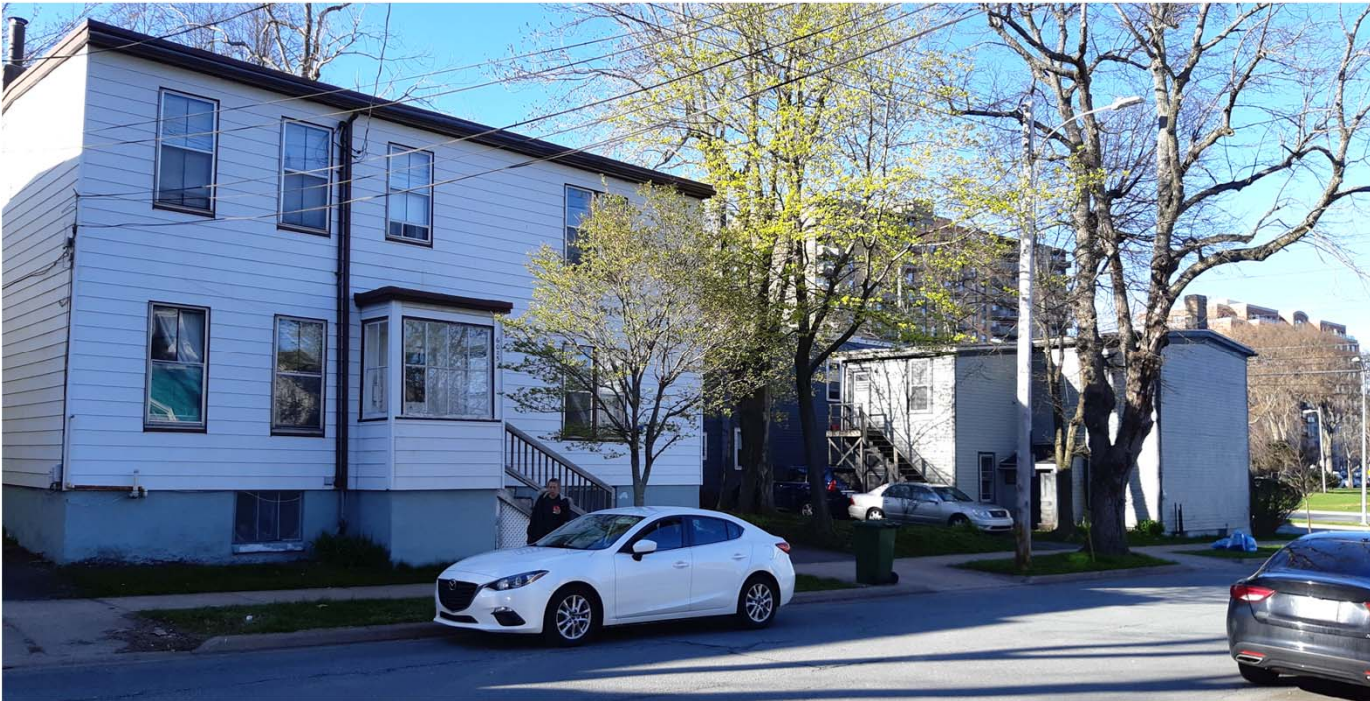
Subject site seen from Compton Avenue
