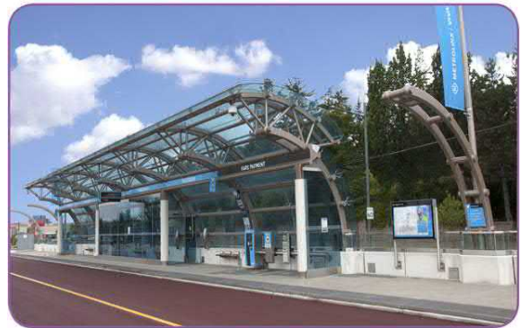
Figure 12: VIVANext Station Platform (York Region)
