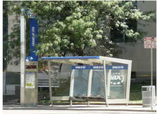
Figure 15: BRT Station Shelter (Kansas City)
