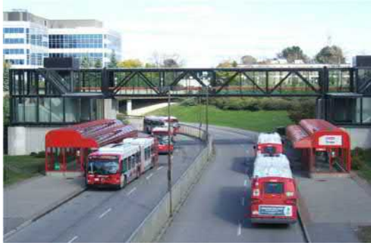
Figure 3: Transit Station in Separate Right-of-Way (Ottawa)
