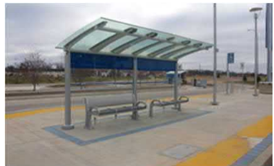
Figure 19: Platform Seating (Winnipeg)
