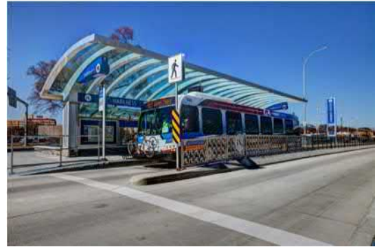
Figure 9: Median Barrier, Platform Railing between Bus Stop and Crosswalk (Winnipeg - Harkness Station)
