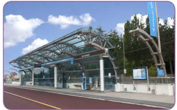
Figure 10: VIVANext Station Platform (York Region)
