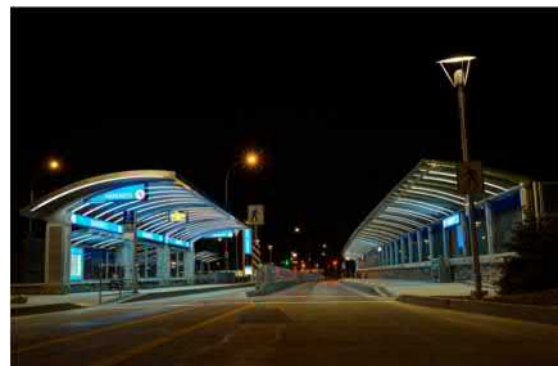
Figure 16: Station Canopy (Winnipeg)
