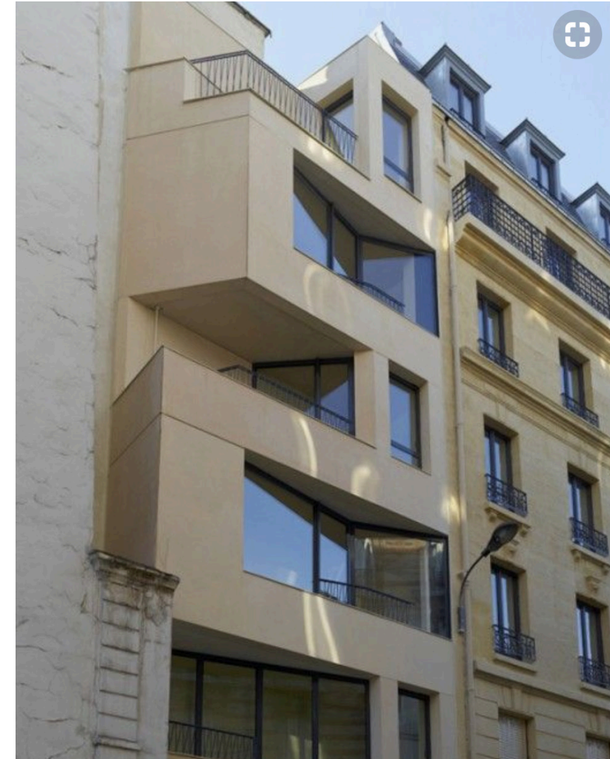
20 SOCIAL HOUSING, H2O ARCHITECTS, PARIS
