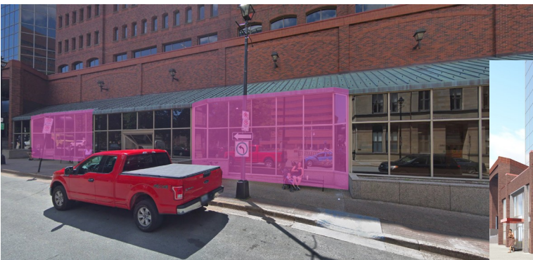
Figure 1. Existing streetwall conditions along Argyle St.
