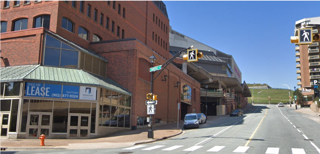
Figure 4. Existing Duke St. blank wall conditions
