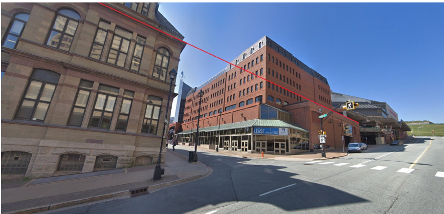
Figure 9. Datum line of Halifax City Hall cornice.
