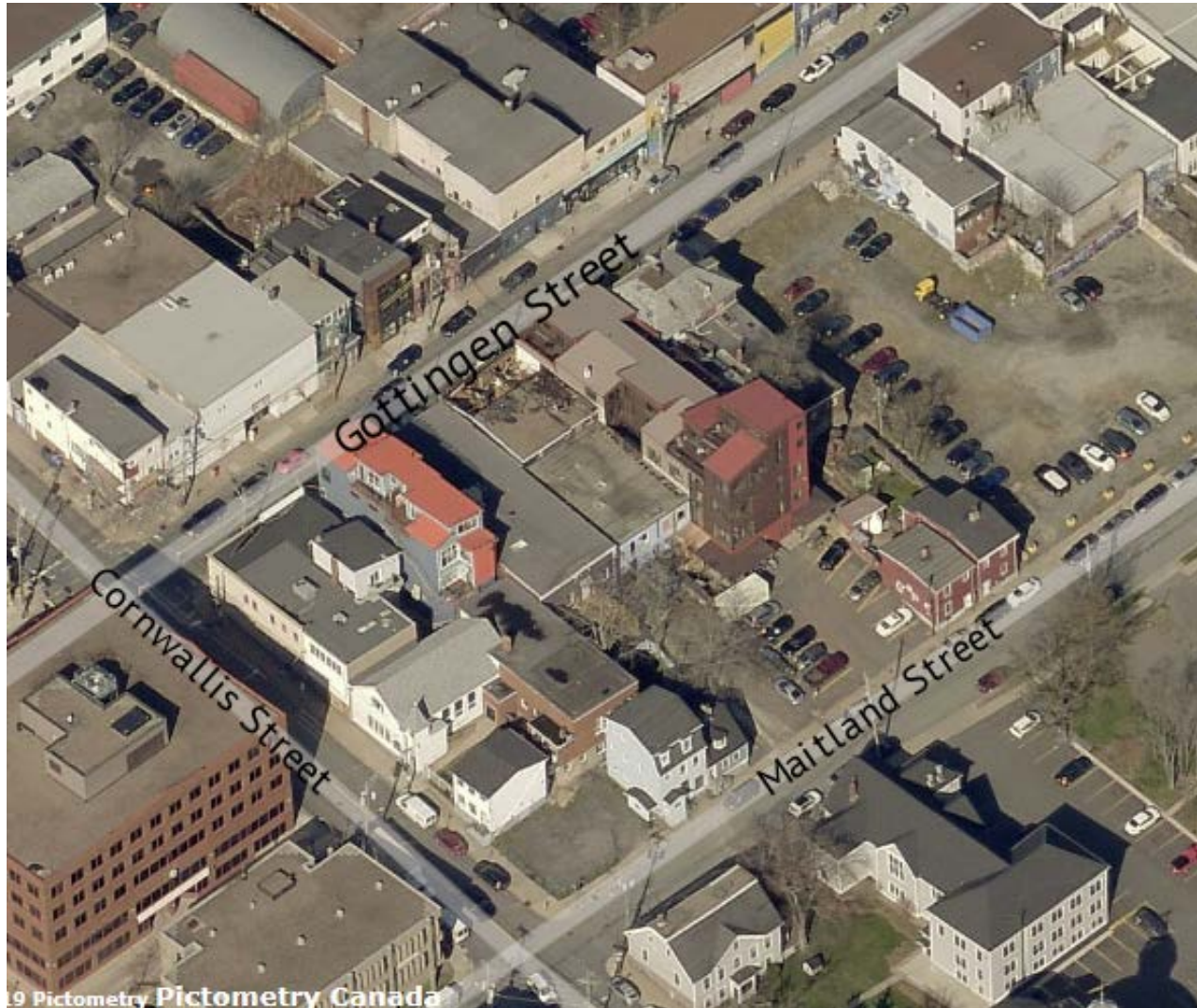
Arial view from SE.
