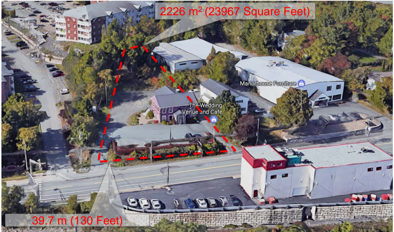
Aerial view of subject site looking west.
