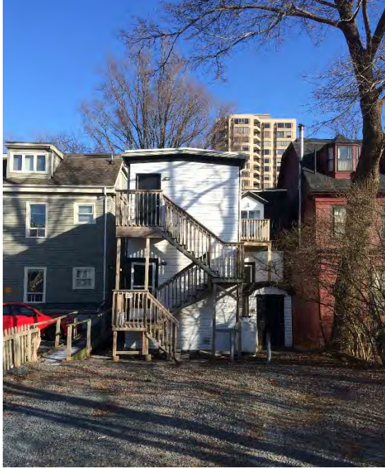
Rear (west) Elevation and Yard
