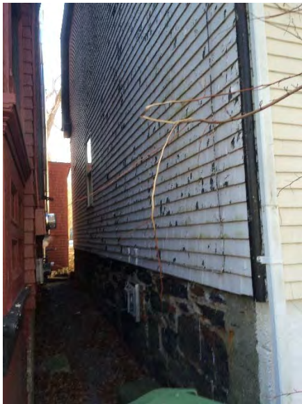
South and North Sidewalls. Note peeling paint shows darker Colour
