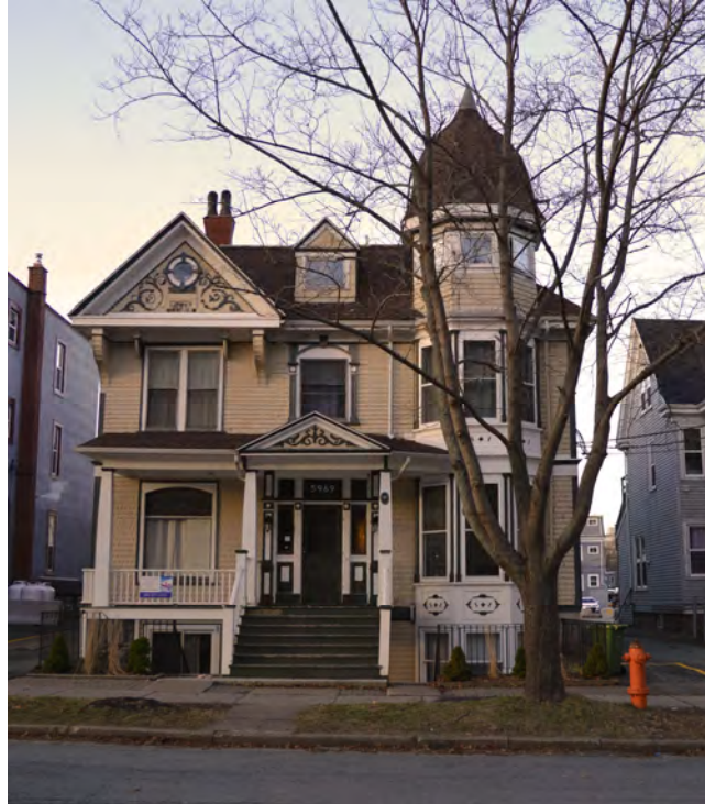
Figure 1. Gold Cure Institute, 5969 College St., photos by Architect.
