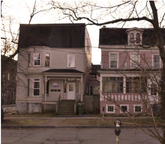
Figure 4. 1452 and 1456 Carlton St. from street Photos by Architect.
