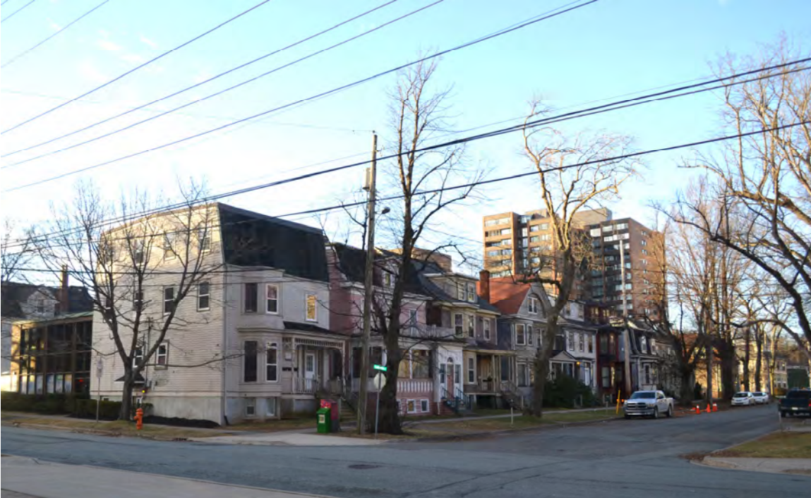
Figure 1. Photo depicting the south west corner of the Carlton Victorian Streetscape, photo by Architect.
