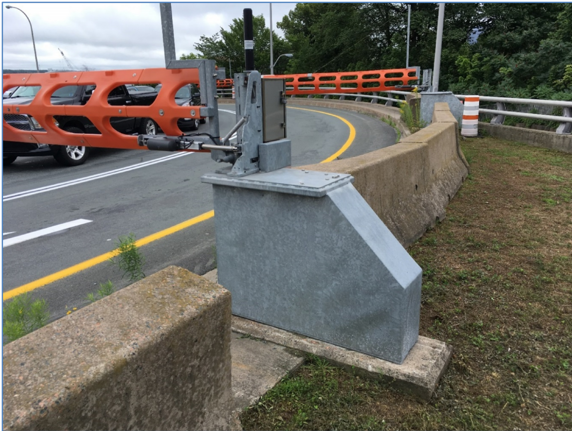
Figure 24 Existing Gates along Outside of Ramp
