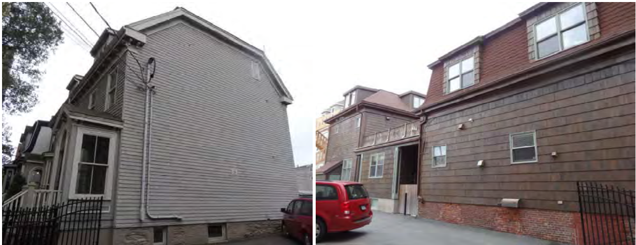
North Wall 1484 Carlton and South Wall 1494 Carlton
