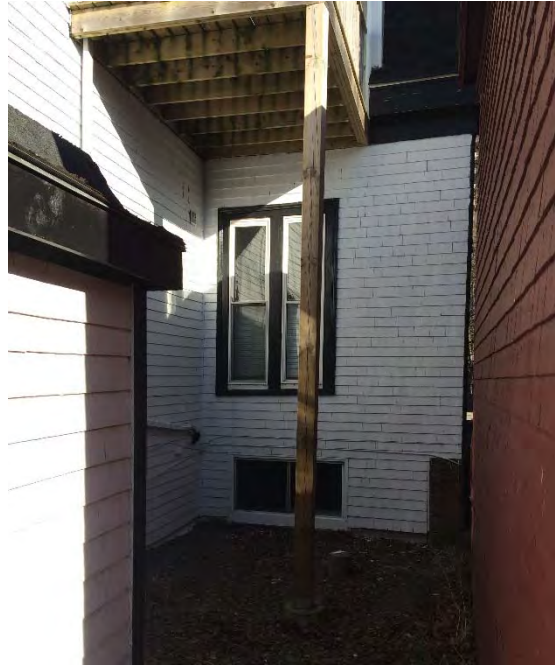
Rear Wall. Note original Window.
