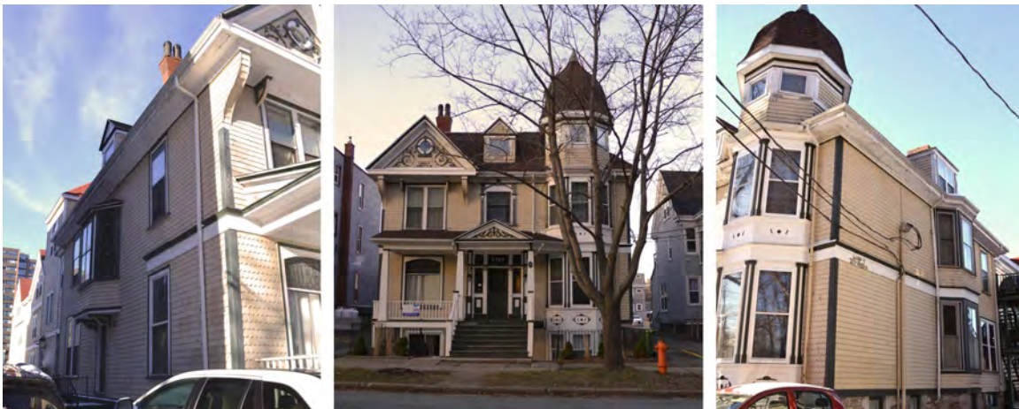
Figure 2. West, South, and East façades Gold Cure Institute, 5969 College St., photos by Architect.
