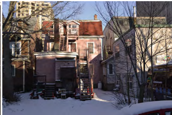
Figure 5. 1452 and 1456 Carlton St. from rear. Photos by Architect.
