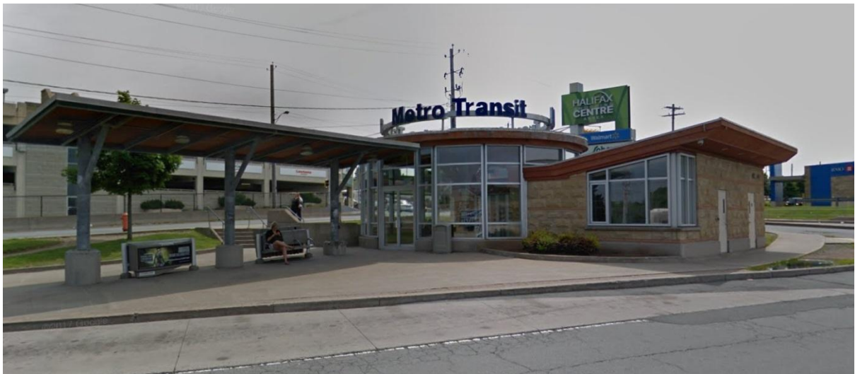
Figure 4: Building and Canopy Area at South End of Mumford Terminal (looking southeast)
