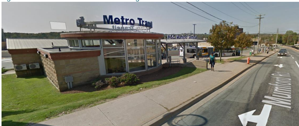
Figure 2: Mumford Terminal - Looking North from East Perimeter Road
