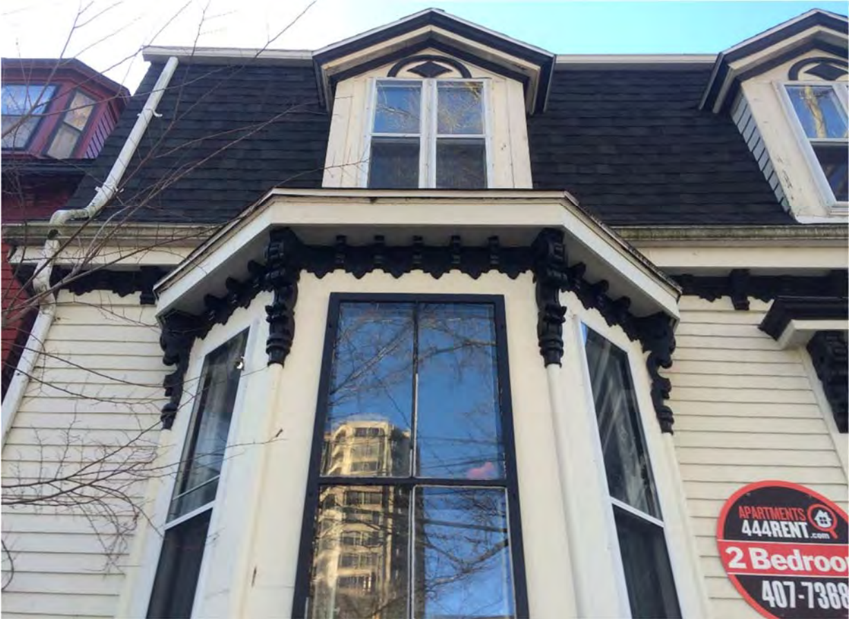
Bay and Entry Door Trim work
