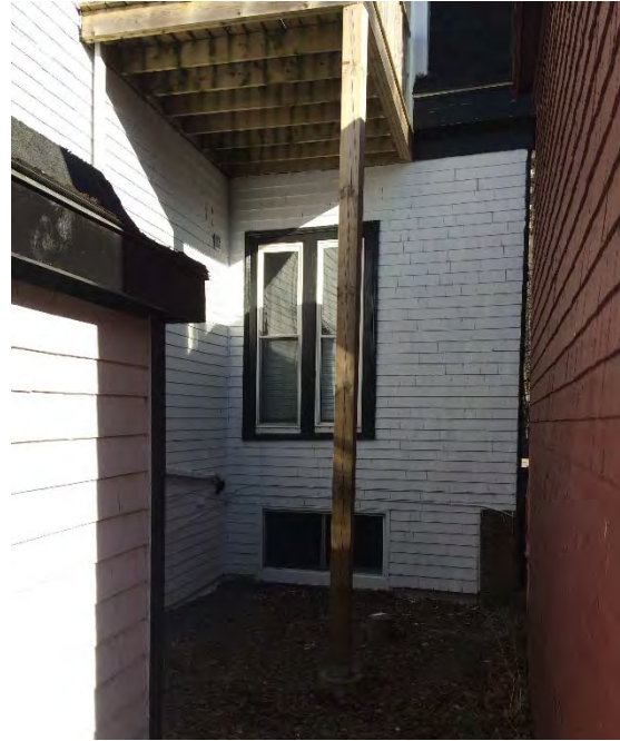
Rear Wall. Note original Window.
