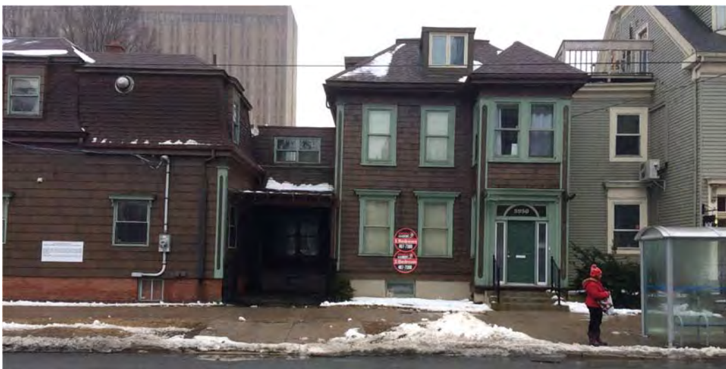
5950 Spring Garden North Elevation with adjoining addition to 1494 Carlton.
