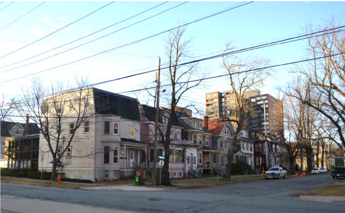
Figure 1. Photo depicting the south west corner of the Carlton Victorian Streetscape, photo by Architect.
