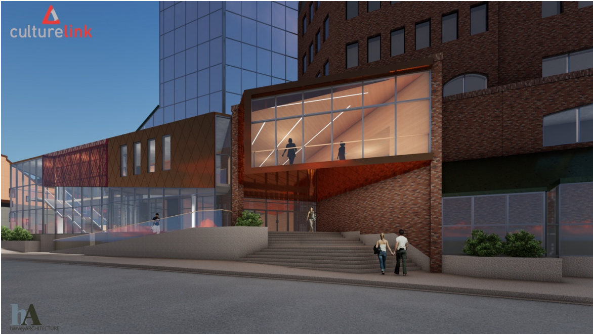
Early stage rendering of The Link, as viewed from Argyle Street Entrance
