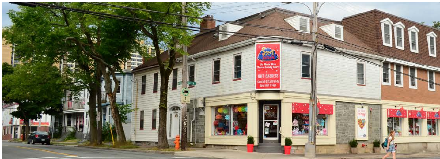
Converted shop front with picture frame windows on a historic Georgian mansion.
