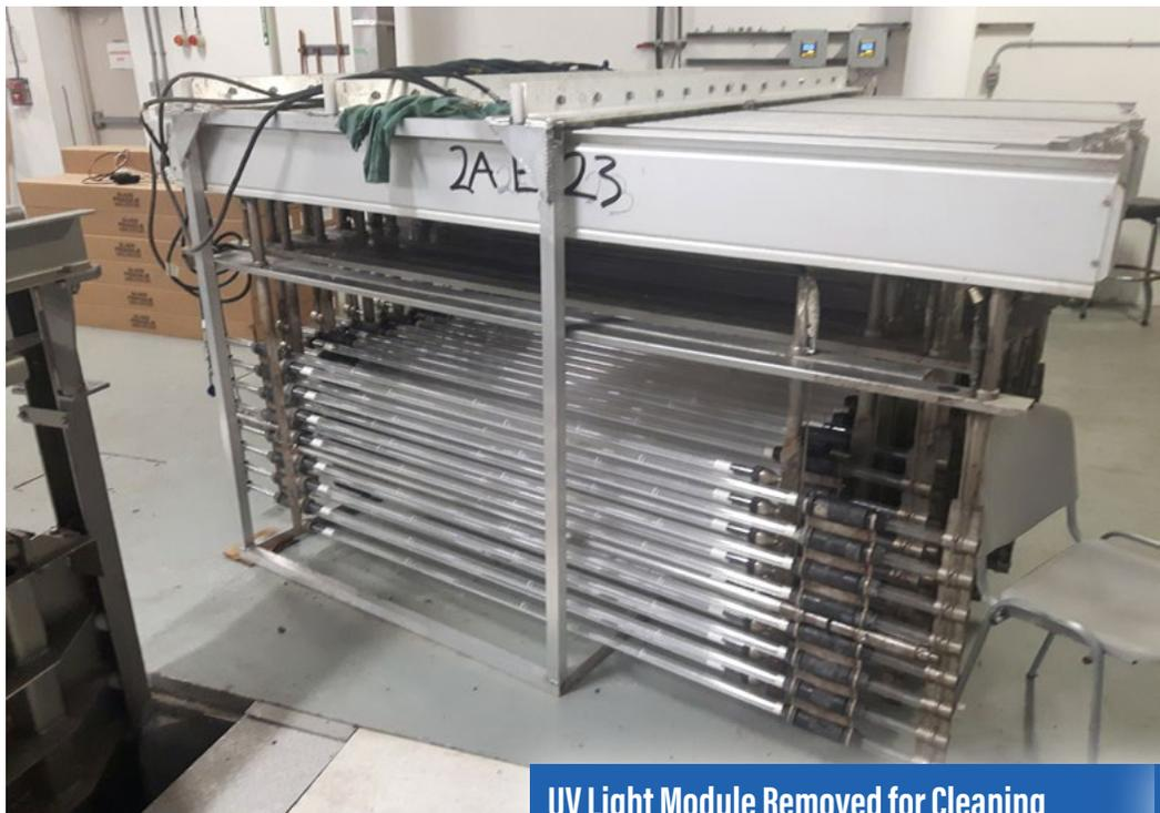
UV Light Module Removed for Cleaning
