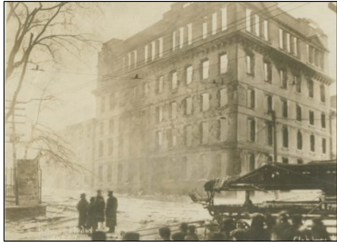
Figure 6: The Kenny-Dennis building showing the shell of the four-storey granite façade topped by the one-storey 1901 addition, shortly after the fire in 1912. Source: NSARM
