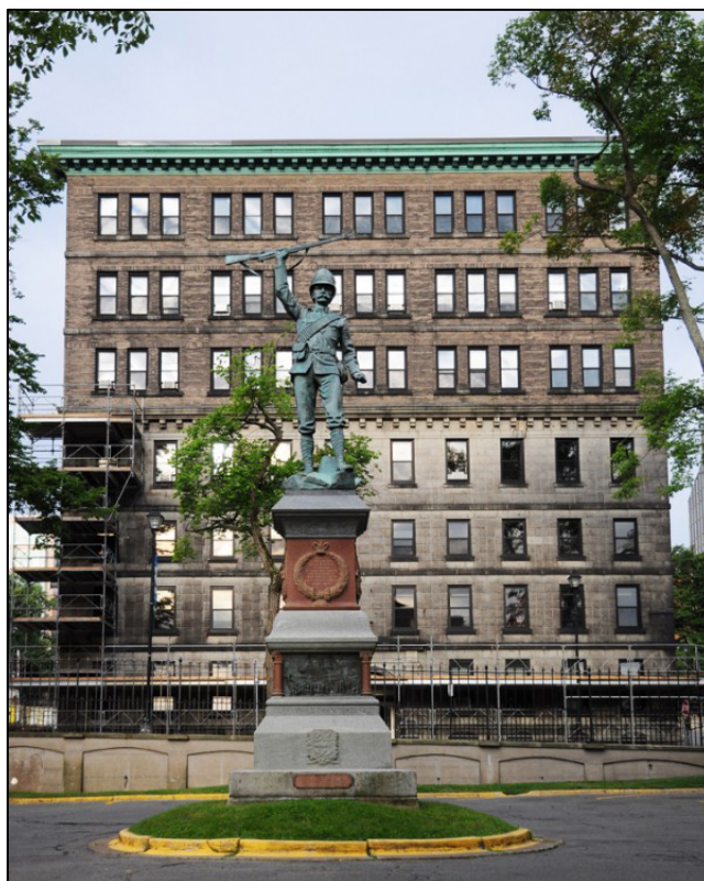
Figure 7: The classically-inspired Kenny-Dennis Building as seen from the grounds of Province House. Photo: Aaron Segart
