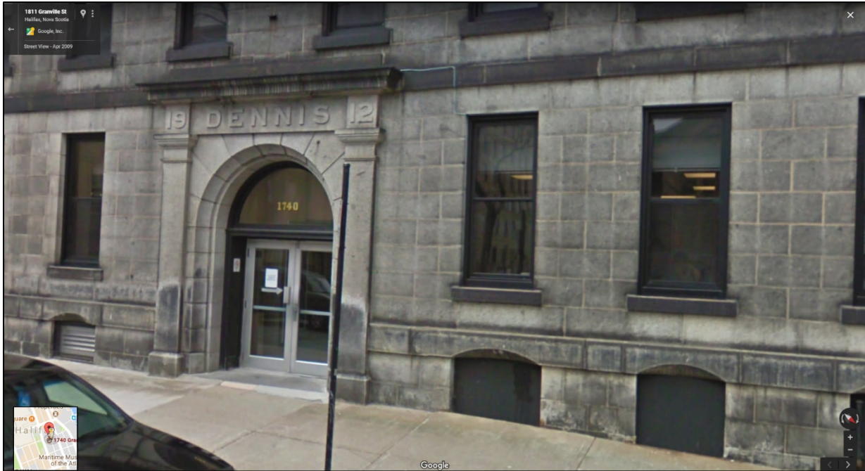
Figure 8: Front facade of the Kenny-Dennis Building showing central arched entrance, dark string course, dark lug sills under the windows, and plinth course with square opening capped by arched carvings in the water table. Source: Google Street View 2009.
