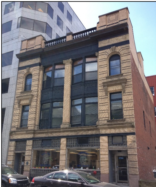
Figure 13: the Beaux Arts style of the Acadian Recorder Building employs a modern approach to the classical theme of the area.
