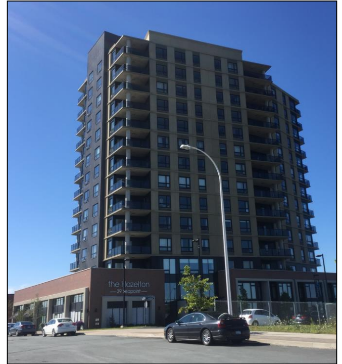
The Hazelton Building (Seapoint Drive)
