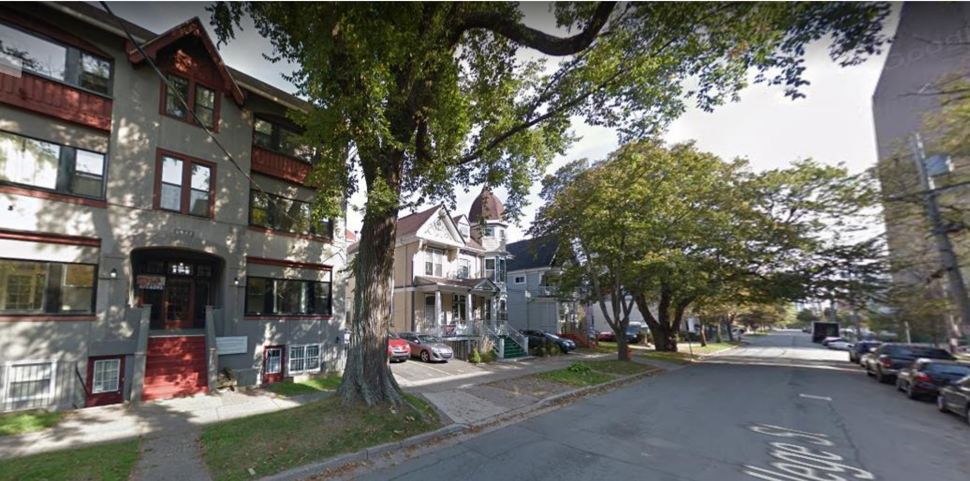
Subject site looking northeast from College Street.
