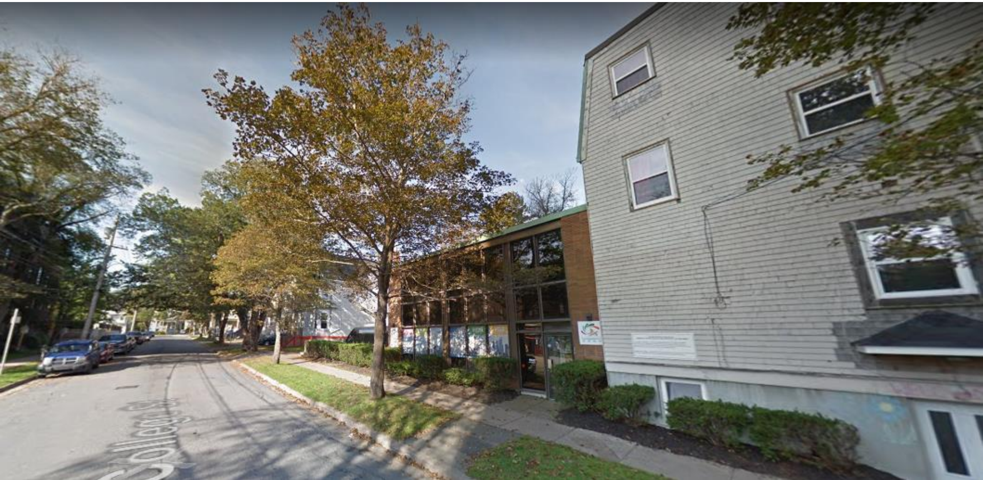
Subject site looking west from College Street.
