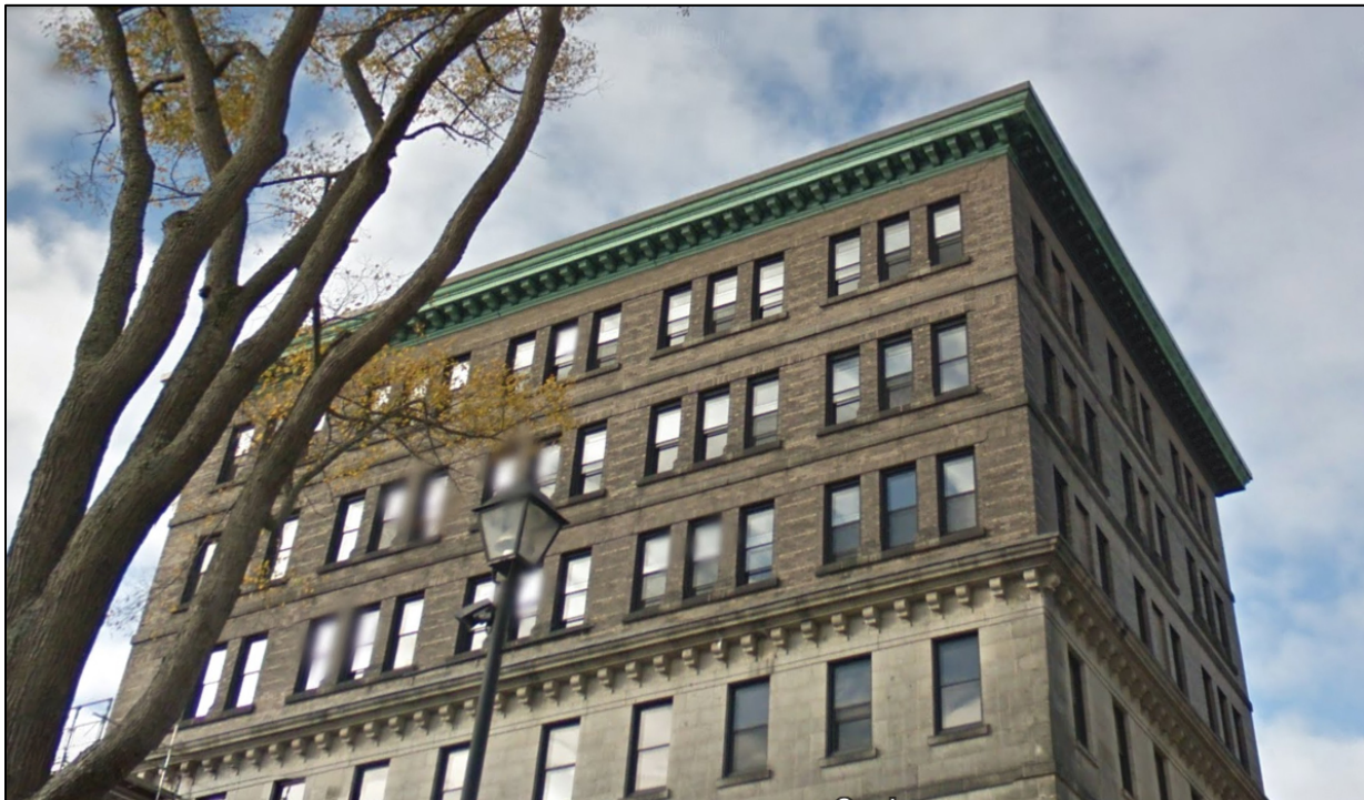
Figure 9: Upper three storeys of the Kenny -Dennis Building showing triplet hung windows within each of five bays on the front façade with strong bracketed cornices above the original granite façades and on top of the brick addition. Source: Google Street View 2012.
