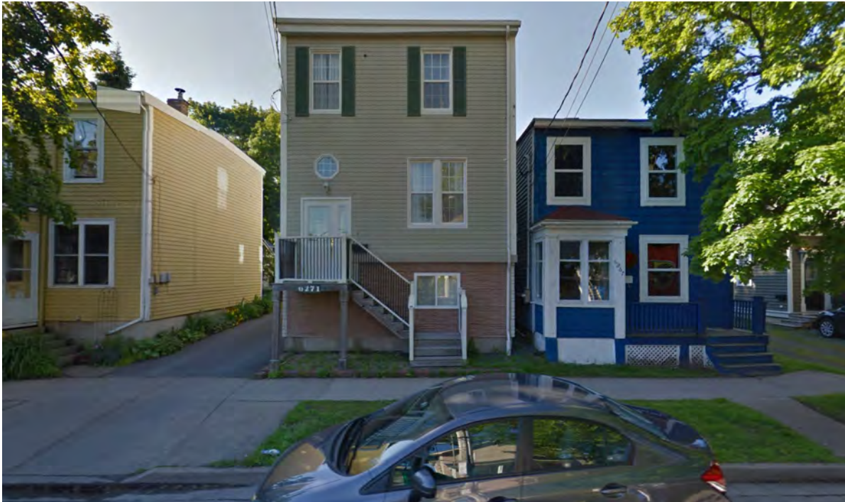
4. #6267 ( on the right in blue) prior to demolition
