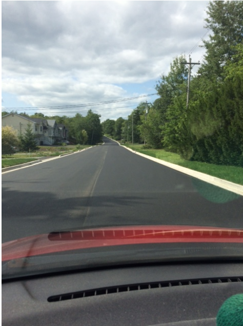
Checking out the recent paving project in the Green Forest Subdivision
