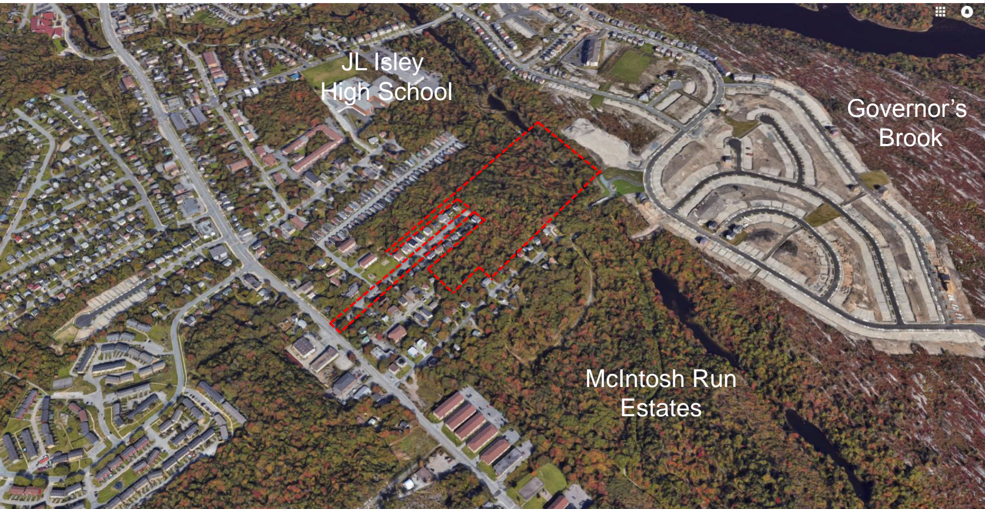
Subject site seen from the south
