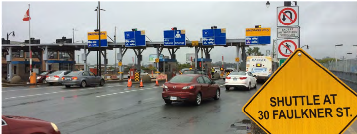
Photo 1 - Looking west on October 6, 2015 toward Macdonald bridge toll lanes from Wyse Road (The centre toll lane is closed)
