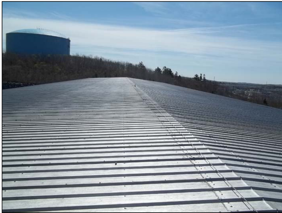
PHOTO 21 - GENERAL OVERVIEW OF RECEIVING AND VESSEL AREA ROOF
