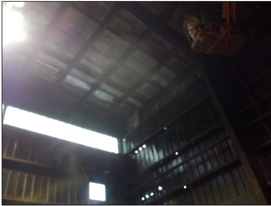
PHOTO 9 - INTERIOR OF SOUTHWEST CORNER WHERE METAL SIDING THAT PREVIOUSLY BLEW OFF HAS BEEN TEMPORARILY PUT BACK IN PLACE WITH PINS
