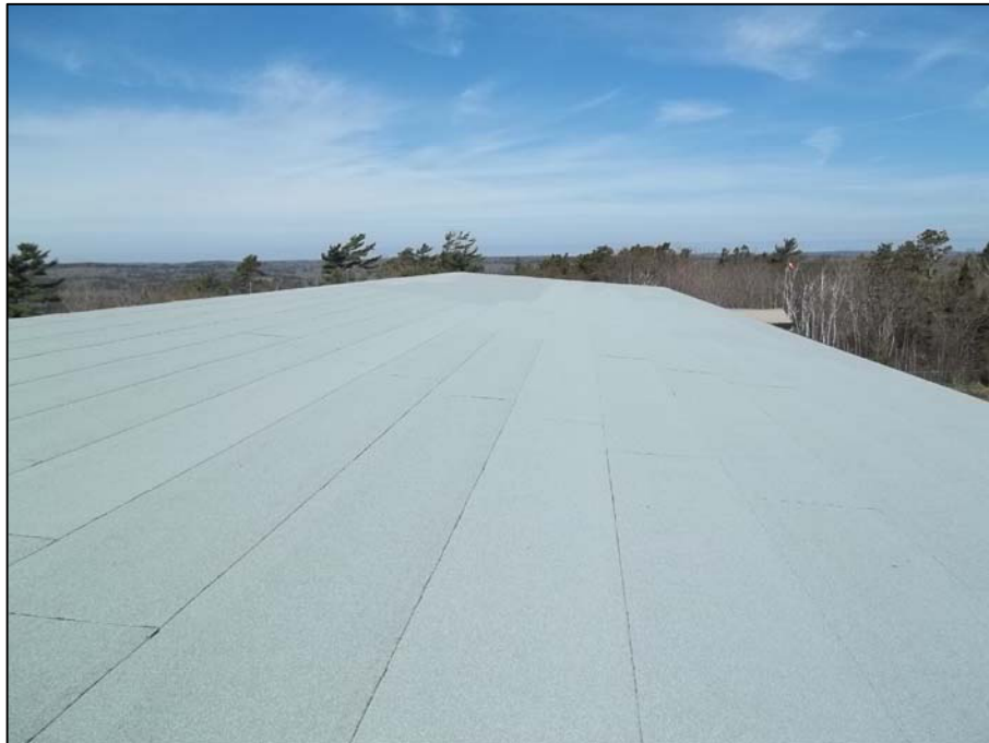
PHOTO 20 - OVERVIEW OF CURING AREA ROOF
