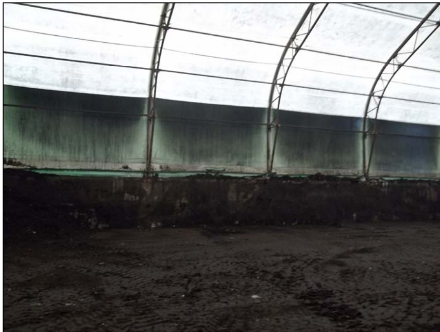
PHOTO 22 - TYPICAL INTERIOR OF FABRIC WALLS OF SCREENING BUILDING
