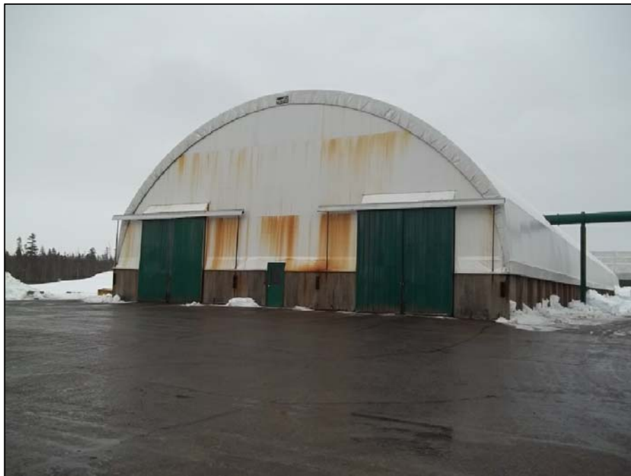
PHOTO 2 - GENERAL OVERVIEW OF CURING BUILDING
