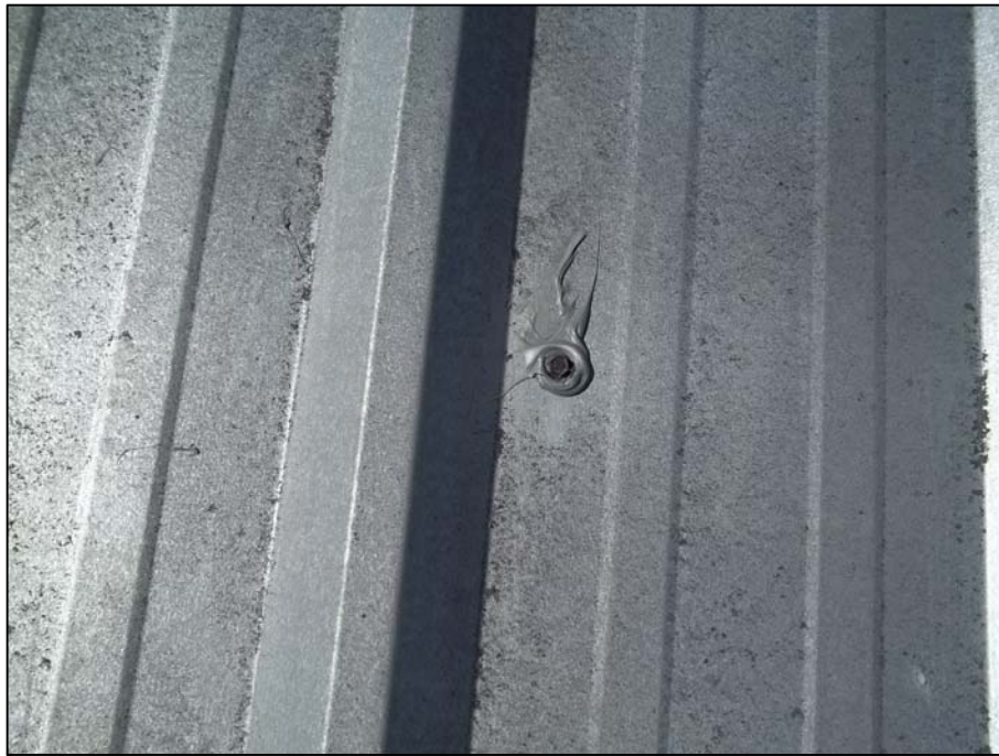
PHOTO 23 - TYPICAL ROOF SCREW THAT HAS BEEN RE-SEALED
