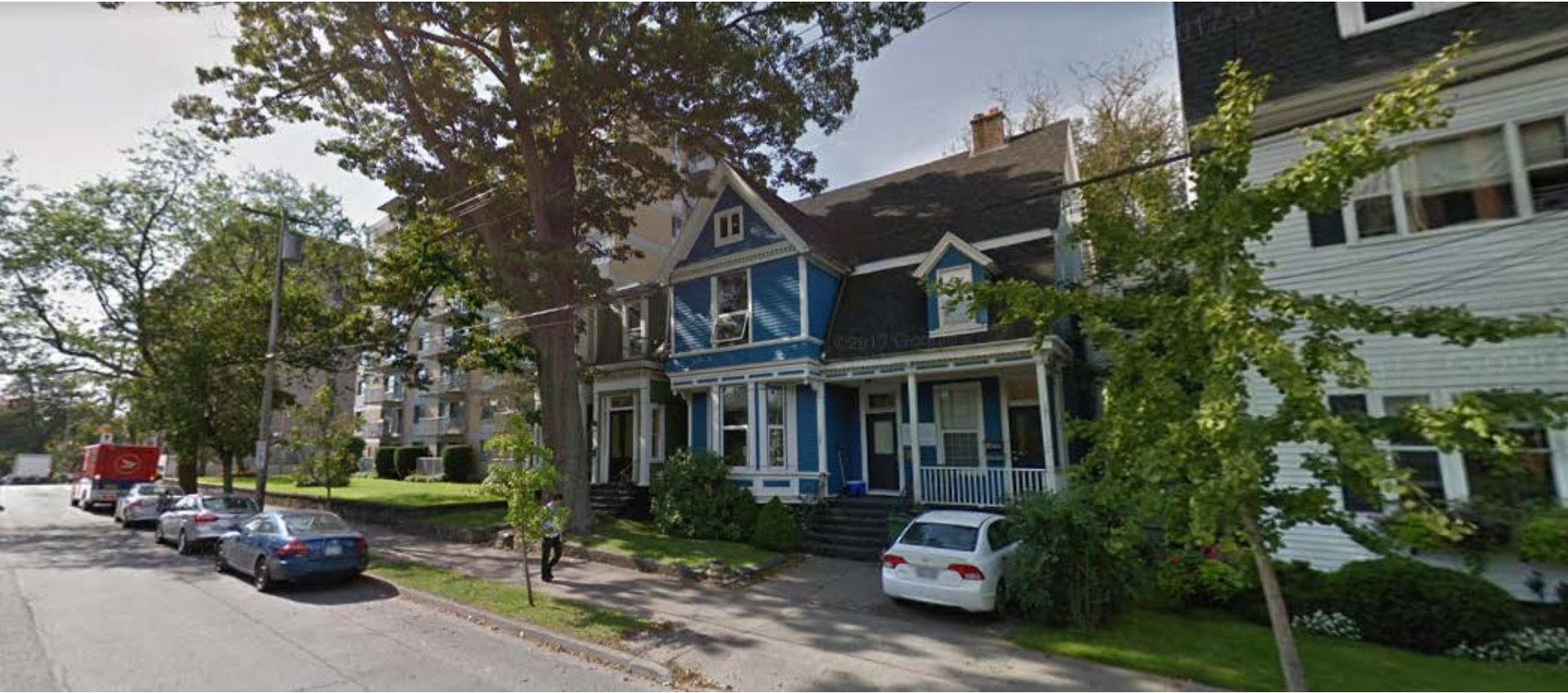
Subject site looking southwest from South Park Street.
