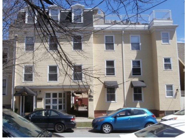
1323-25 Dresden Row (the old bakery) which has been converted into apartments
