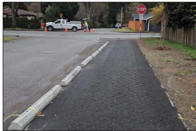
Figure 6: Temporary Sidewalk Installation in Seattle, Washington
