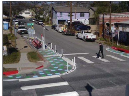
Figure 2: Pedestrian Improvements by Painting Roadway and Adding Bollards
