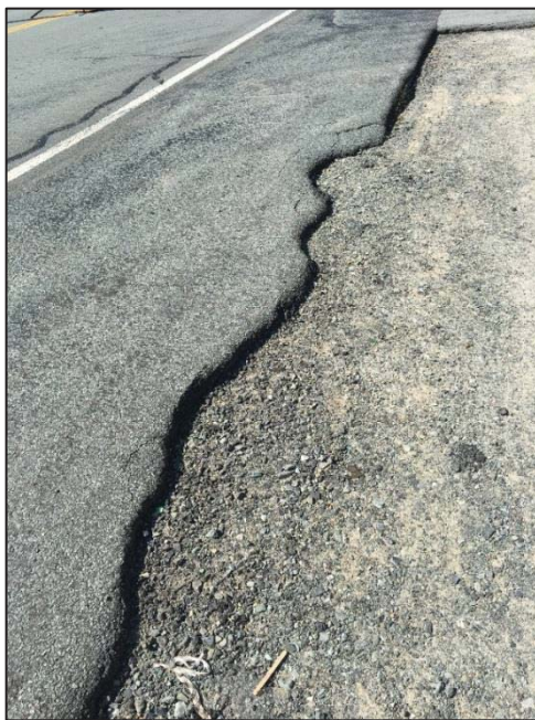
Figure 3: Inconsistent Shoulder Width Sept 2017
