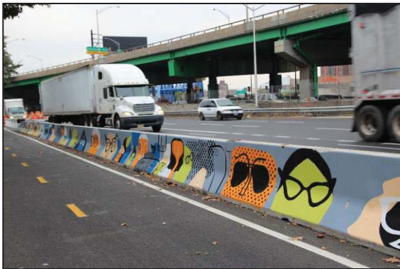
Figure 1: Painted Jersey Barrier on Highway
