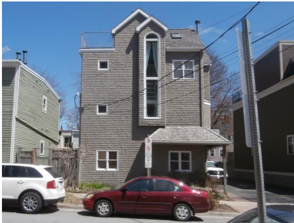
1345 Dresden Row - runs horizontal (vertical?) to street and would look nicer if there were at least one door facing the street
