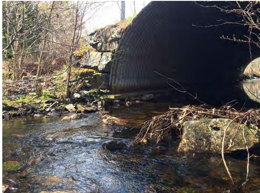
Photo 9: KL2 Kearney Lake Sample Location (lake side of culvert)
