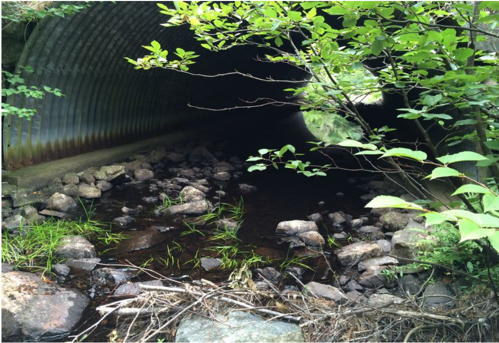
Photo 9: KL2 Kearney Lake Sample Location (lake side of culvert)
