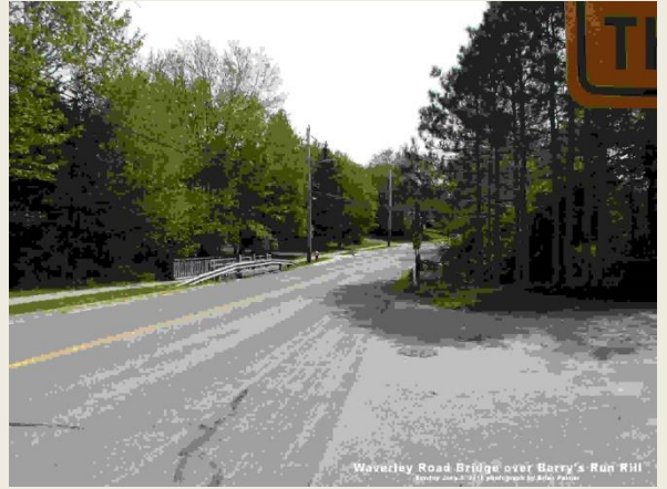
Waverley Road Bridge over Barry's Run RMI Sunday June 3, 2018 photograph by Brian Palmer
