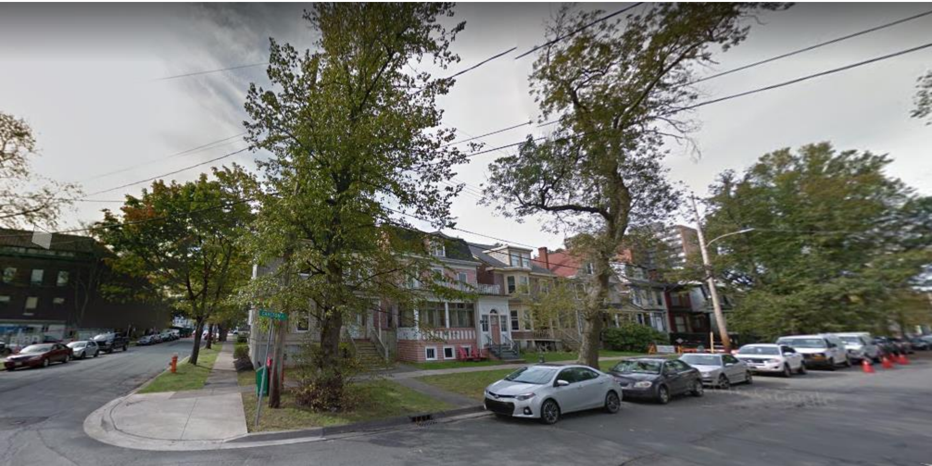
Subject site looking west from Carlton Street.
