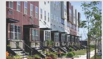
2 Street-facing residential units reflect traditional Halifax row houses with a contemporary flair, and can form the lower floors of mid-rise or mixed use buildings.
