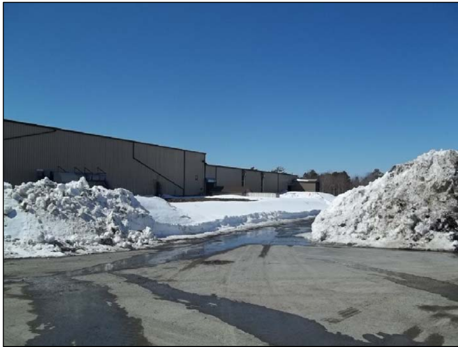
PHOTO 1 - GENERAL OVERVIEW OF NORTH ELEVATION
