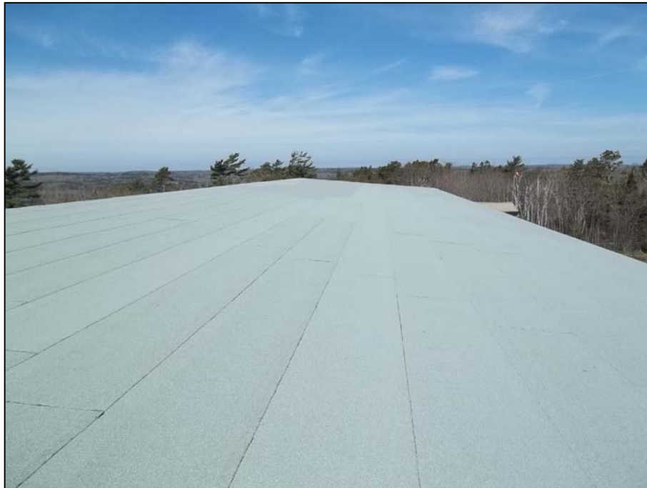
PHOTO 20 - OVERVIEW OF CURING AREA ROOF
