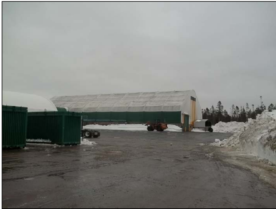
PHOTO 3 - GENERAL OVERVIEW OF SCREENING BUILDING
