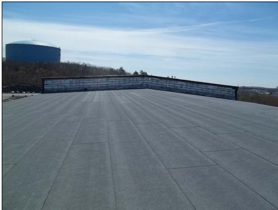
PHOTO 22 - WALL AT JUNCTION OF HIGH ROOF AND LOW ROOF WITH ONLY TYVEK AIR BARRIER
