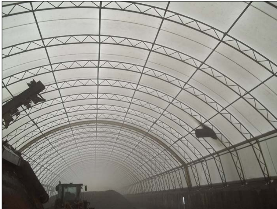
PHOTO 16 - INTERIOR OF CURING BUILDING
