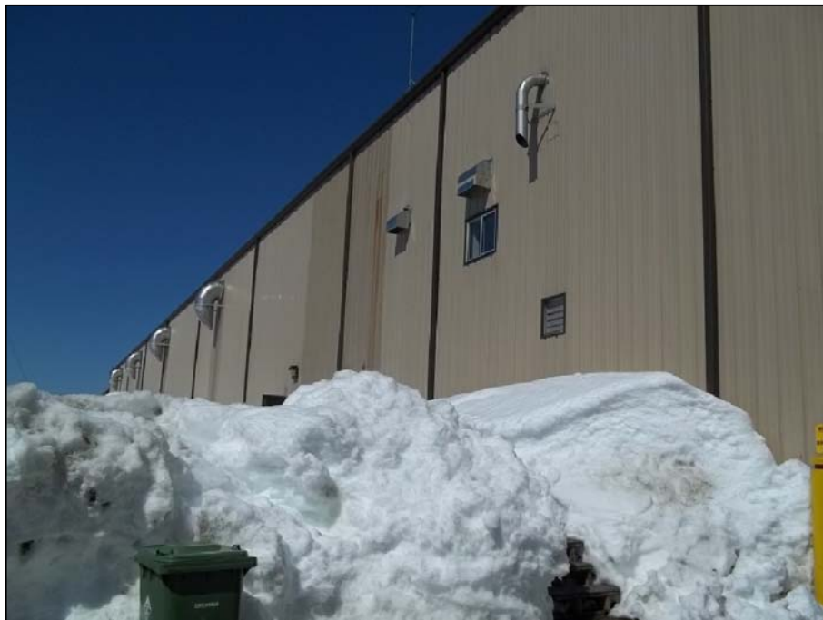
PHOTO 2 - GENERAL OVERVIEW OF SOUTH ELEVATION
