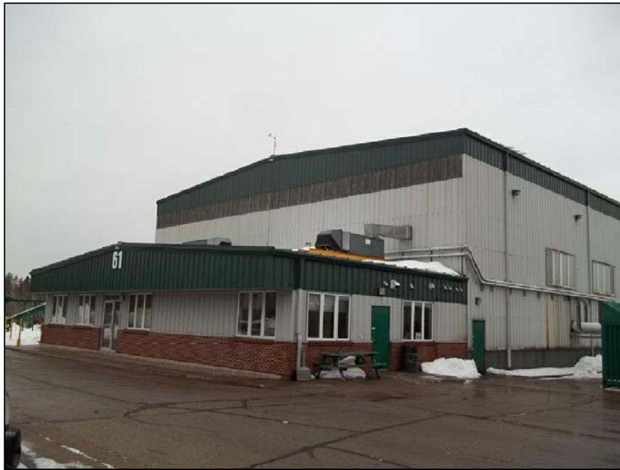
PHOTO 1 - SOUTH ELEVATION OF OFFICE AND RECEIVING BUILDING
