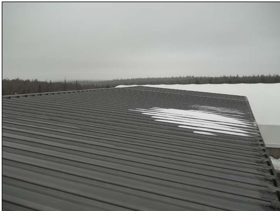
PHOTO 4 - GENERAL OVERVIEW OF ROOF OF RECEIVING BUILDING
