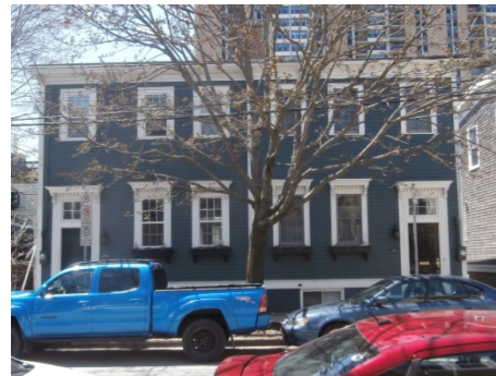
Two-and-a-half storey mirror image houses with shared flat roof on Dresden Row
