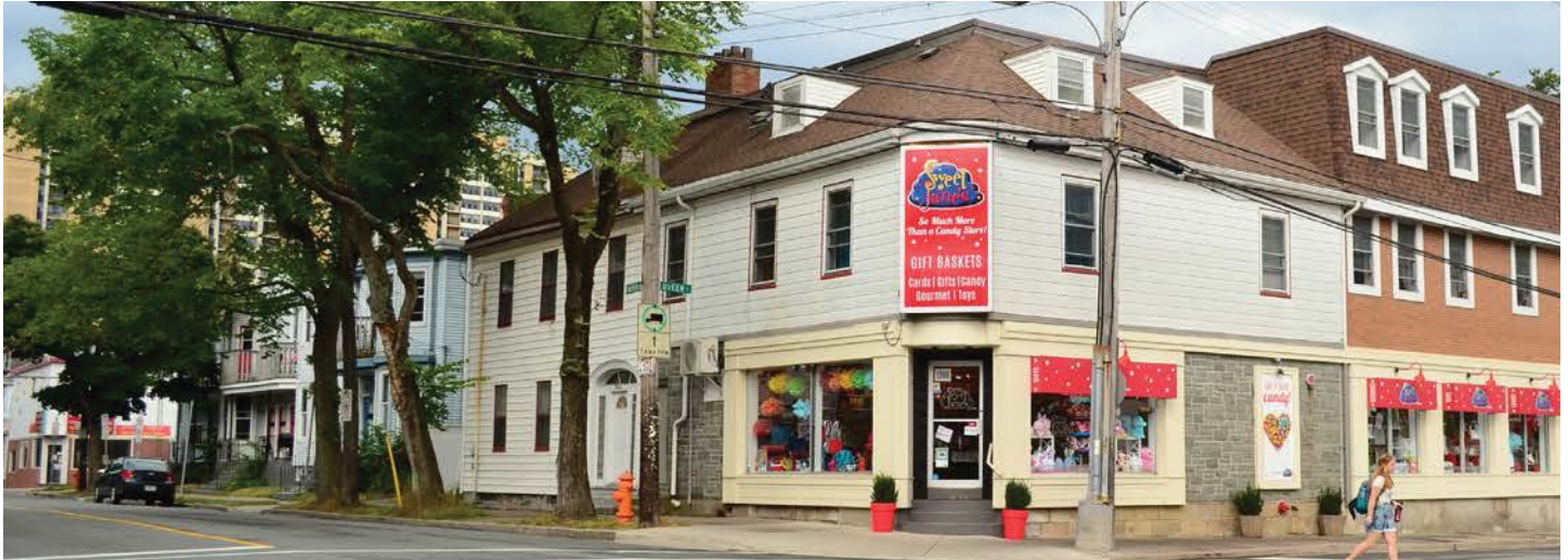
Converted shop front with picture frame windows on a historic Georgian mansion.
