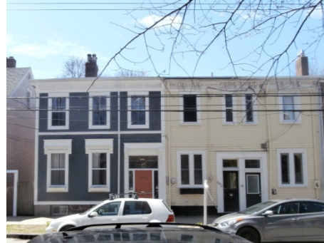
Building, on left, with decorative hood moldings over windows and doors.
