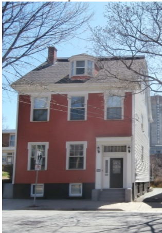
Detached “Halifax House” on Morris Street with truncated gable roof and Scottish dormer
