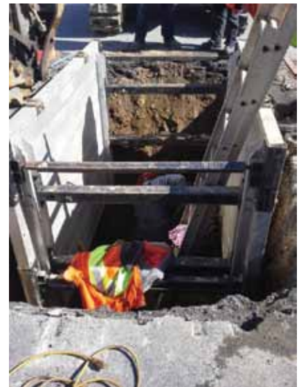
Using a trench box to ensure safe working conditions
