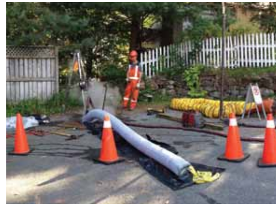
Rehabilitating the Crescent Avenue sewer using innovative trenchless technology
