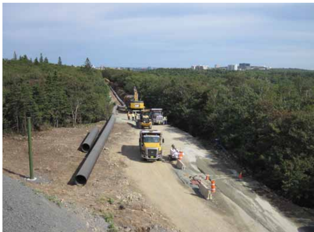
Installation of Sanitary Sewer along the Chain of Lakes Trail
