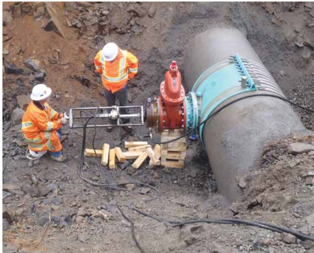
Critical “Hot Tap” of the Pockwock watermain for service to Bedford
