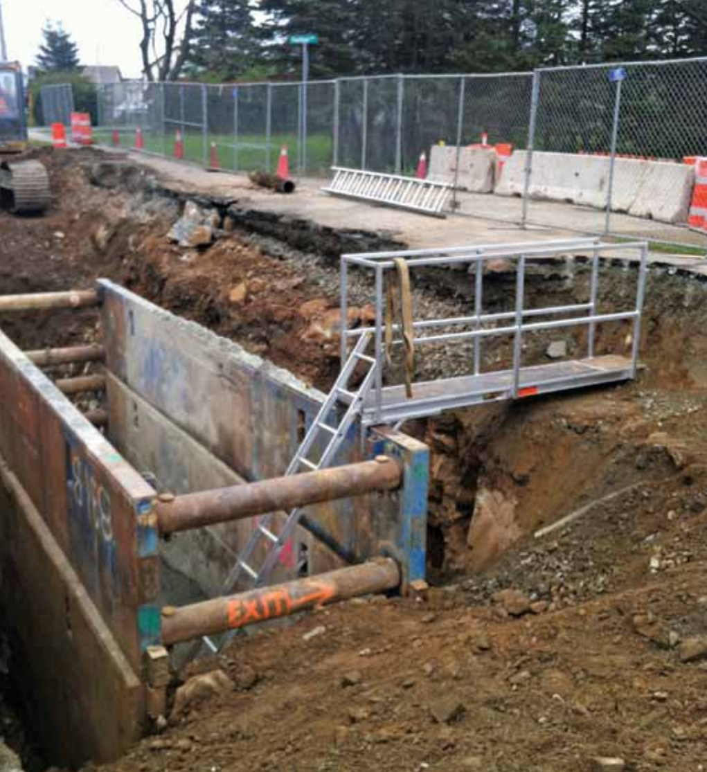
Safety first on the Cow Bay Road deep storm sewer project
