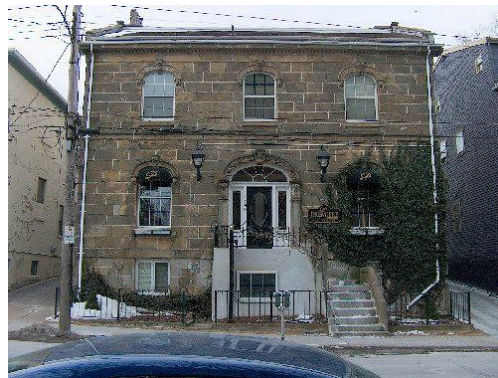
One of only two masonry buildings in the District
