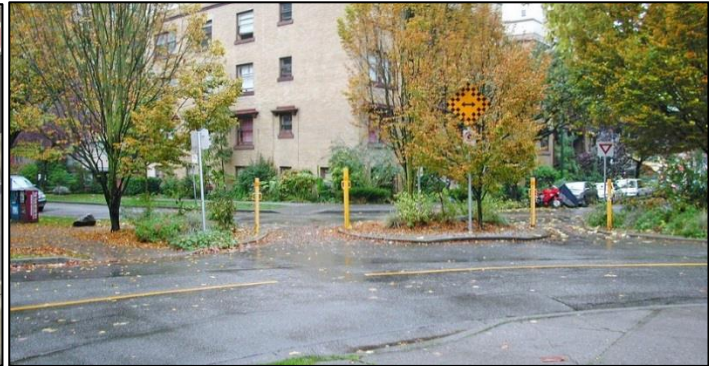
Figure 5: Photo of Diagonal Diverter in Victoria BC
