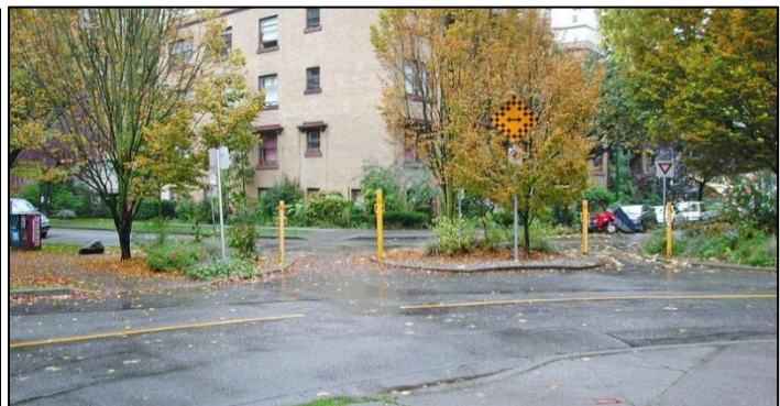
Figure 7: Photo of Diagonal Diverter in Victoria BC
